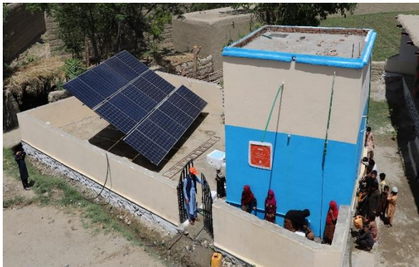
Figure 1 ORCD Successfully completed Construction of SPW
